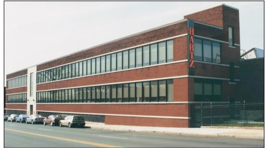
Image of one of the buildings on the Hartz Mountain Site when in full operation.
