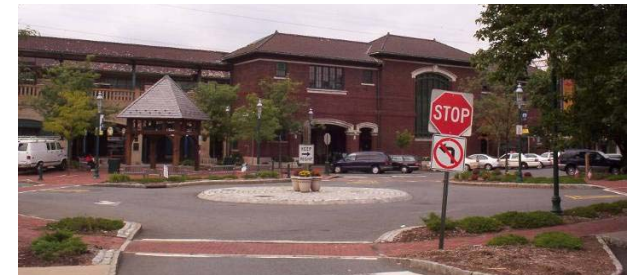
Roundabout, South Orange, N.J.
