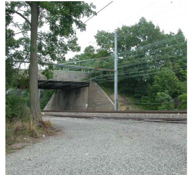
View from the railroad tracks of the Route 571 Bridge
