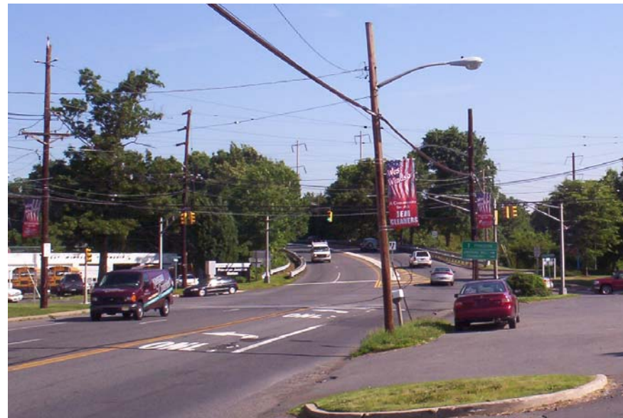
View looking west of the Route 571 Bridge
