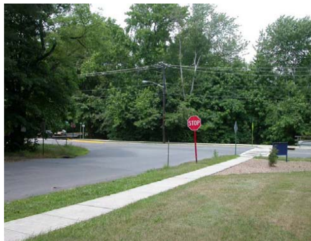
View looking west along Scott Avenue
