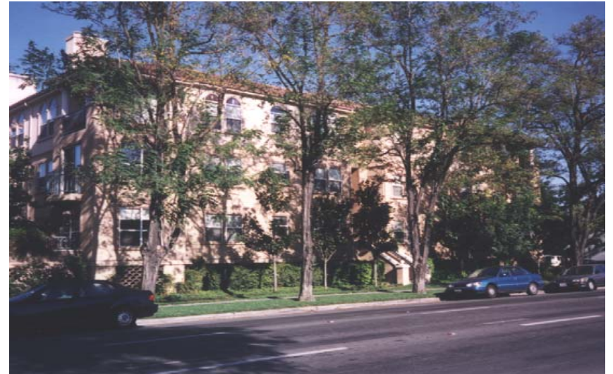
Low-rise residential building over a parking garage, San Jose, Cal.
