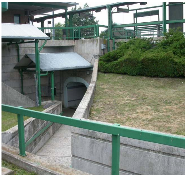
View of the primary pedestrian tunnel ramp
