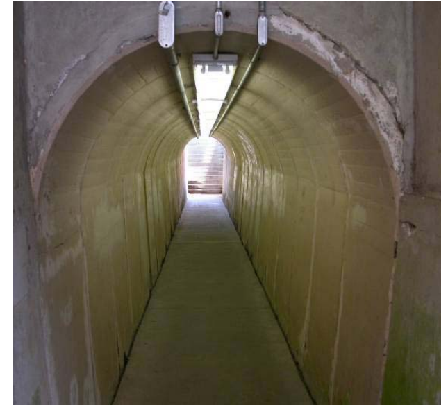
View of the secondary pedestrian tunnel
