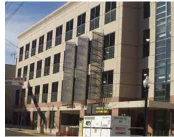
Parking garage, Princeton, N.J.
