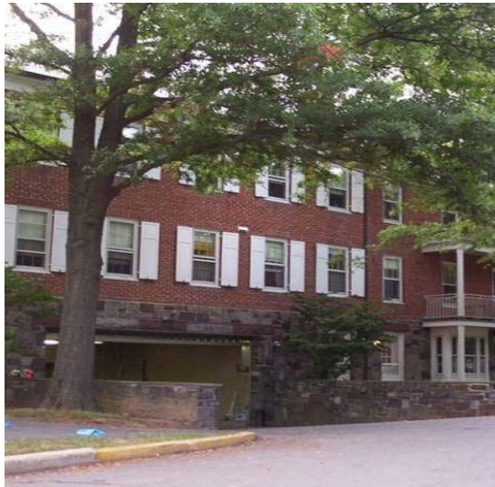
Low-rise residential buildings over a parking garage, Princeton, N.J.
