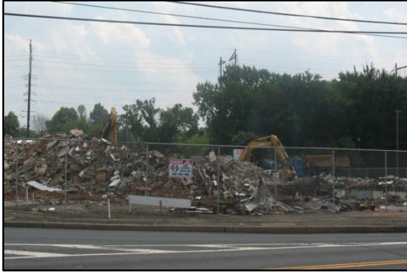
Figure 33: Demolition of former supermarket
