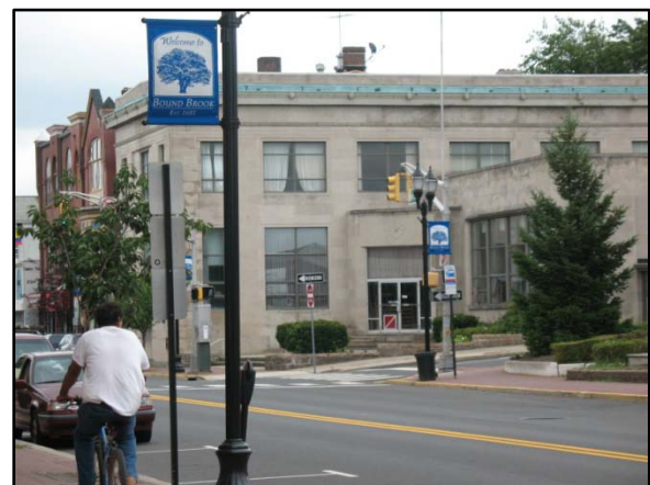
Figure 11: Unoccupied bank Adjacent to the NJ Transit station
