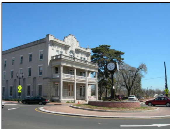
Figure 10: Traffic circle (round-a-bout) North end of Bound Brook's downtown
