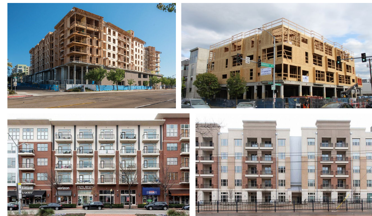
Figure 11. Examples of Podium Construction
